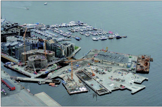
34. Teren budowy Tjuvholmen Museum . Źródło: http://www.skyscrapercity.com/showthread.php?t=765974&page=41 34. The construction site of Tjuvholmen Museum. Source: http://www.skyscrapercity.com/showthread.php?t=765974&page=41
